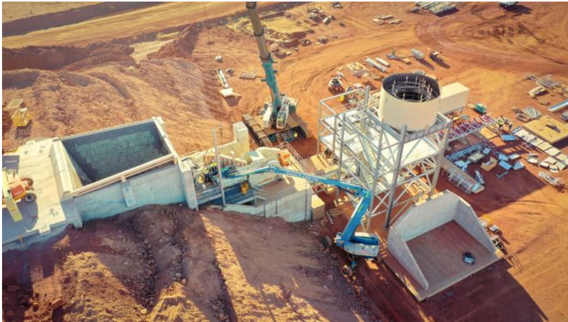
Installing primary crusher steelwork and equipment
