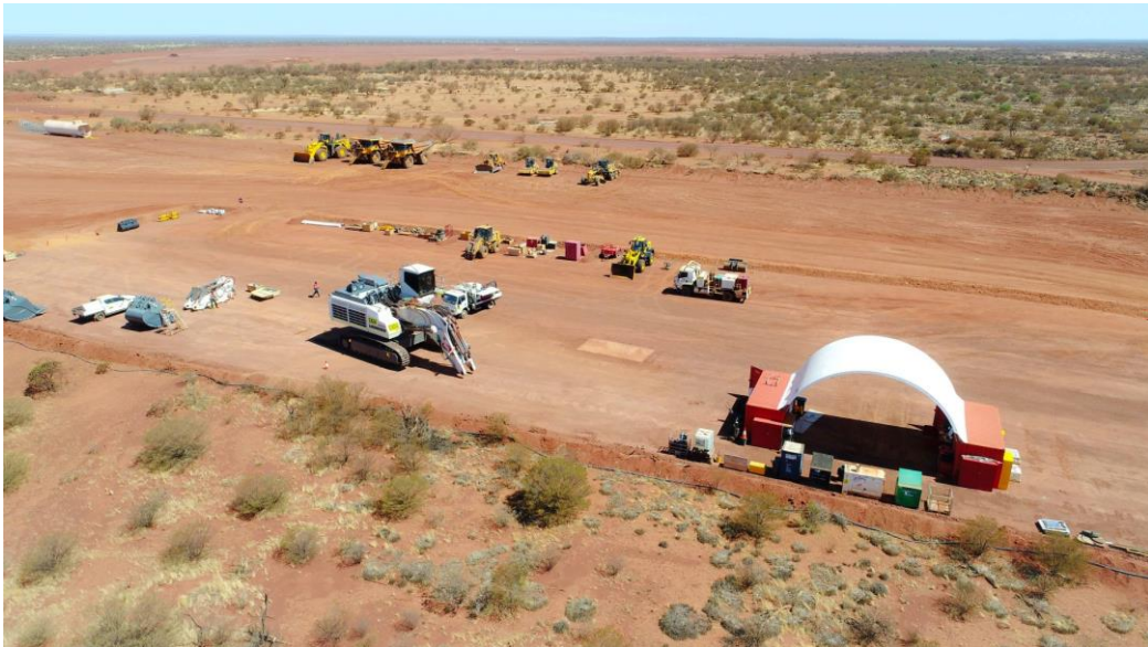
Mobilisation of mining contractor
