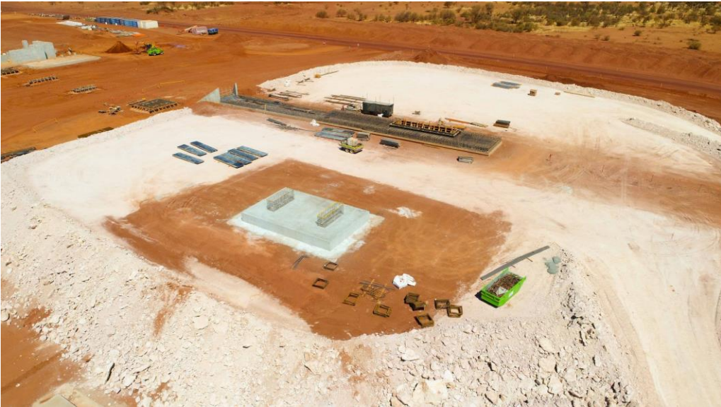
Fine ore stockpile and reclaim tunnel
