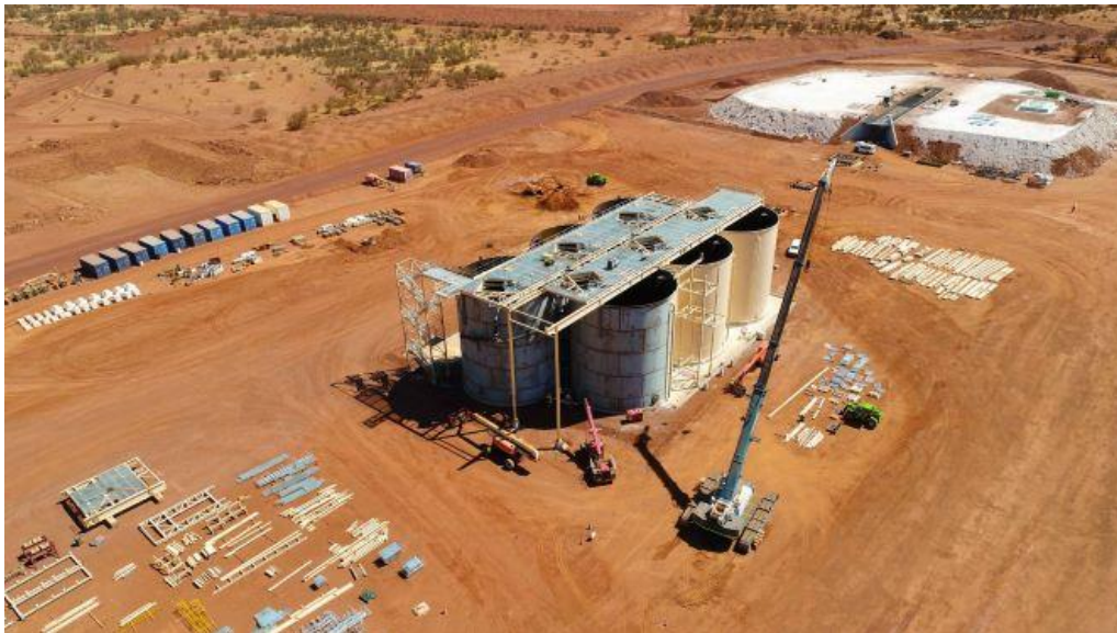
CIL tank erection and top of tank steel installation
