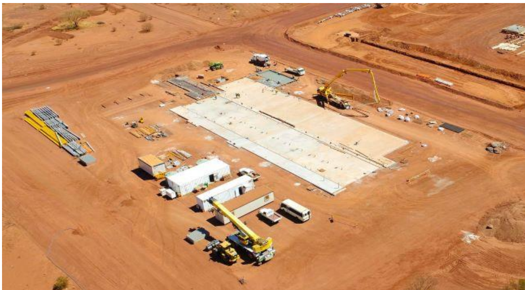
Foundations for power station
