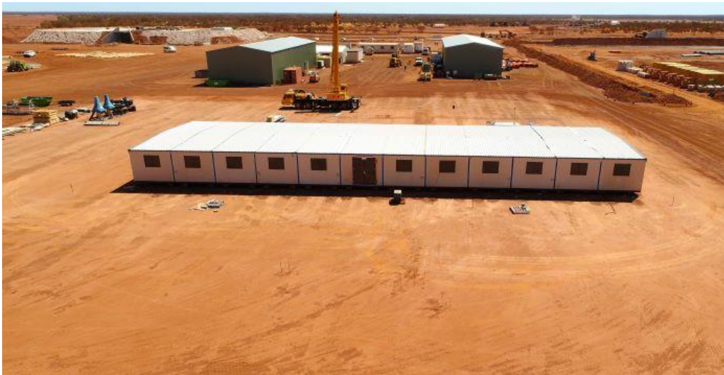
Administration office, Maintenance workshop and stores shed
