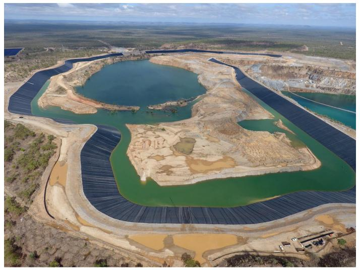
Figure 3: Status of Wises Dam liner placement as at1st December 2023
