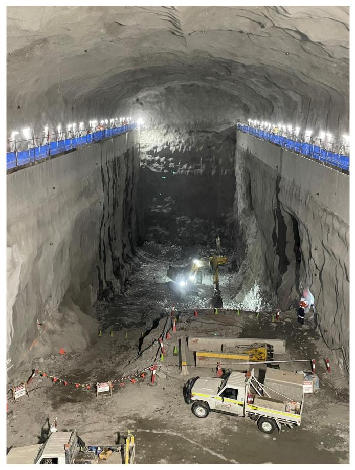
Figure 1: Powerhouse Cavern excavation
