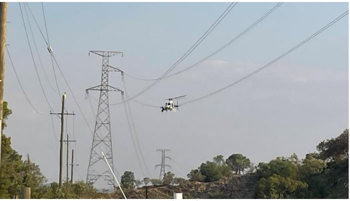
Figure 3: Transmission Line conductor installation finalisation from helicopter (Kidston end)
