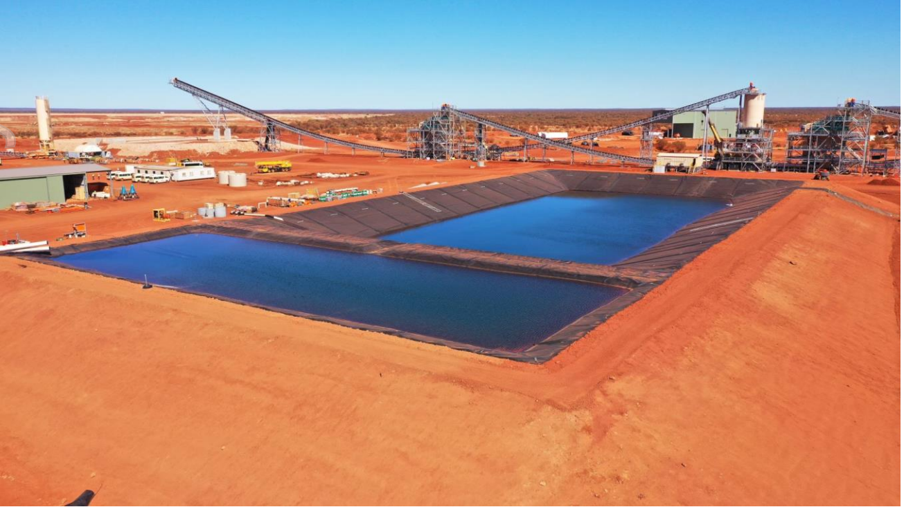
Process water dam
