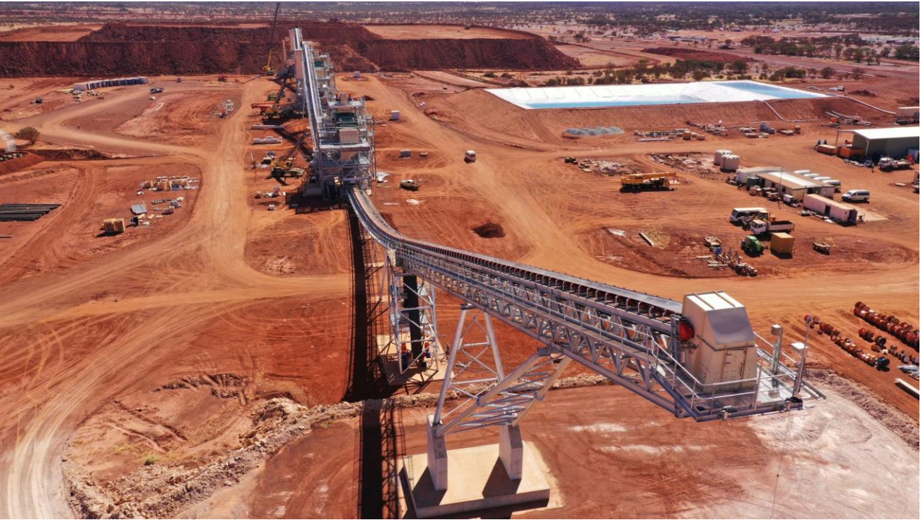
Crushing circuit and ROM
