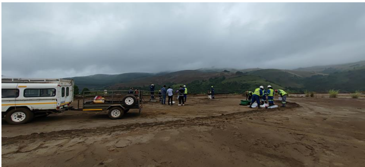
Figure 1 – Drilling by the SGS team being conducted on the main TGME DSF
