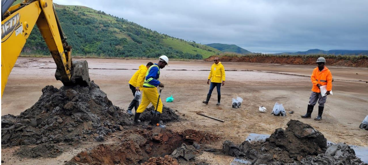
Figure 5 – Sampling at the main TGME DSF adjacent to the TGME Processing Plant completed by YRC’s team
