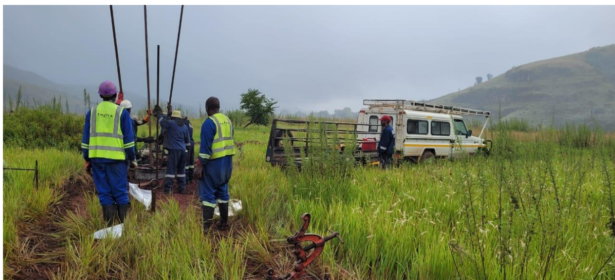
Figure 2 – Drilling by SGS at the Blyde #2 tailing near the TGME plant.
