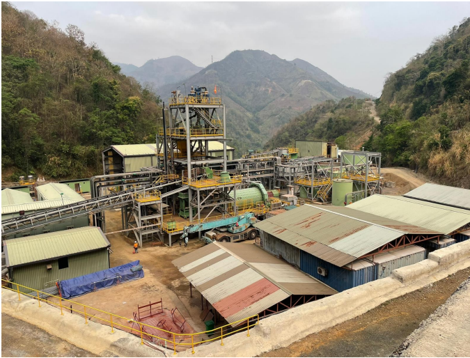
Figure 4: Infrastructure: 450ktpa Nickel Concentrator
