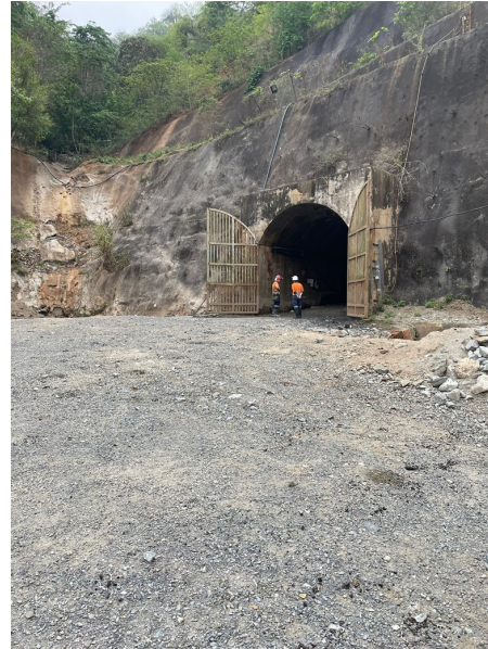
Figure 5: Infrastructure: Underground Portal
