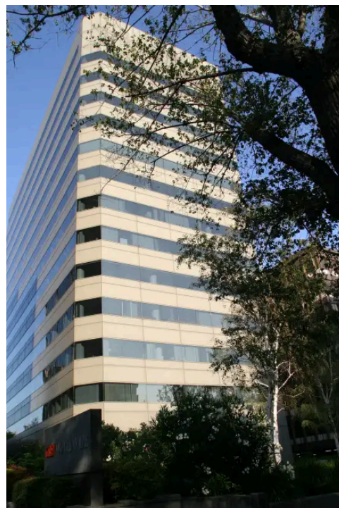
The Australian Unity Office Fund's portfolio includes this office block on Melbourne's St Kilda Road. Michele Ferguson
