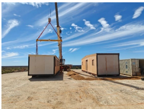
Plate 1: Installation of the Apollo Hill Development Camp
