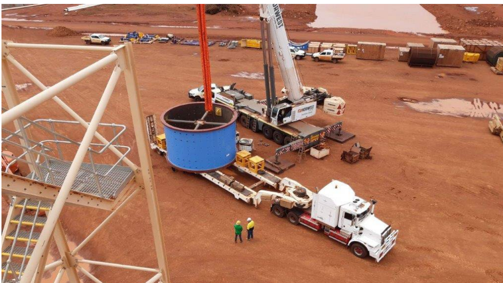
Ball mill oversize loads being delivered to site
