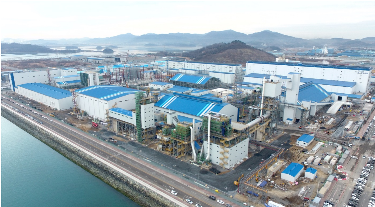
Figure 1: The PLS LHM facility as at 17 January 2024.
