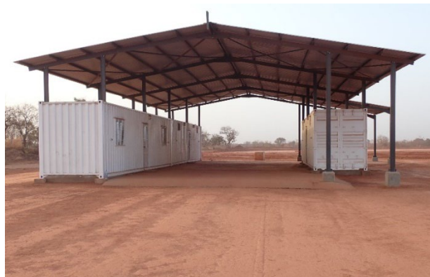
Image 12: New core yard facility
