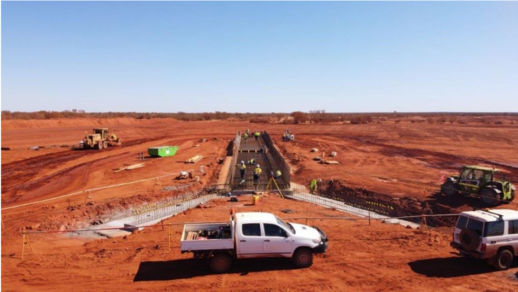
Fine ore stockpile tunnel concrete footing
