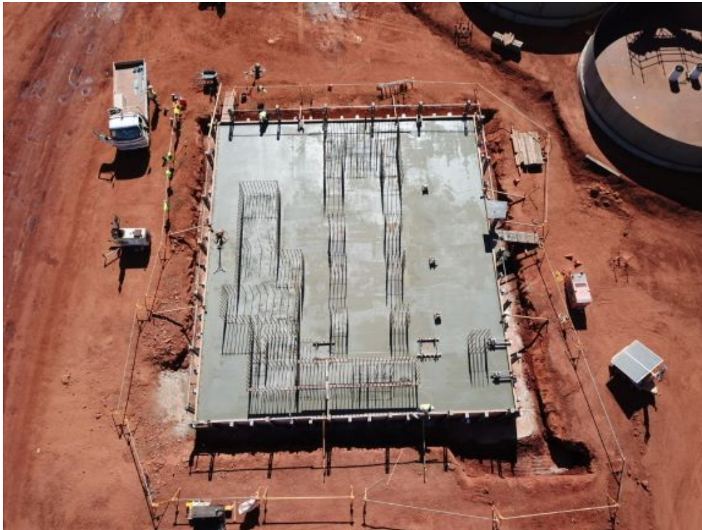
Ball mill foundations
