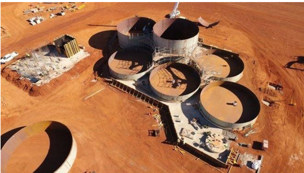
Concrete foundations for ball mill and CIL tank construction
