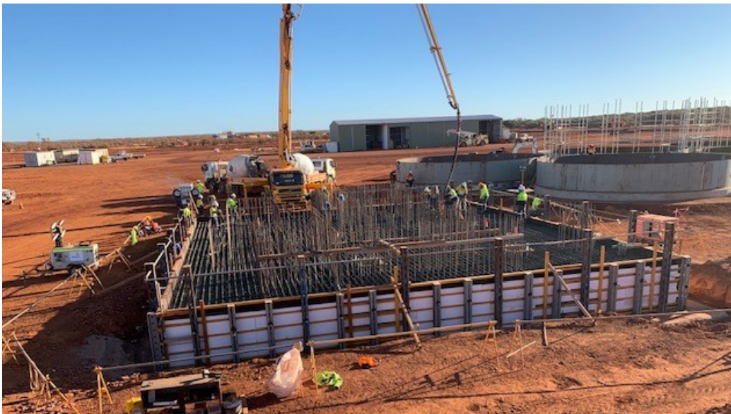
Pouring of concrete foundation for ball mill
