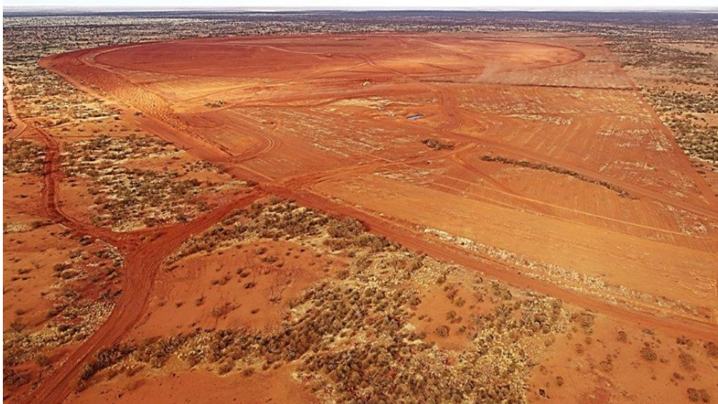
Clearing and topsoil removal for the TSF/IWL
