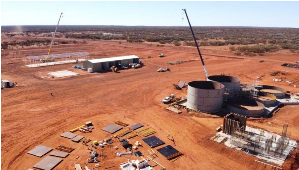
Processing plant construction progress
