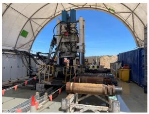
Figure 2: Raisebore Machine Excavating Ventilation Shaft
