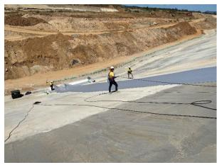
Figure 6: Installing the Geotextile Layer below the HDPE Liner
