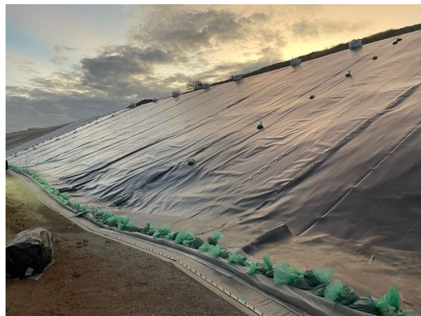
Figure 6: First installation of the HDPE Liner on the Wises Dam
