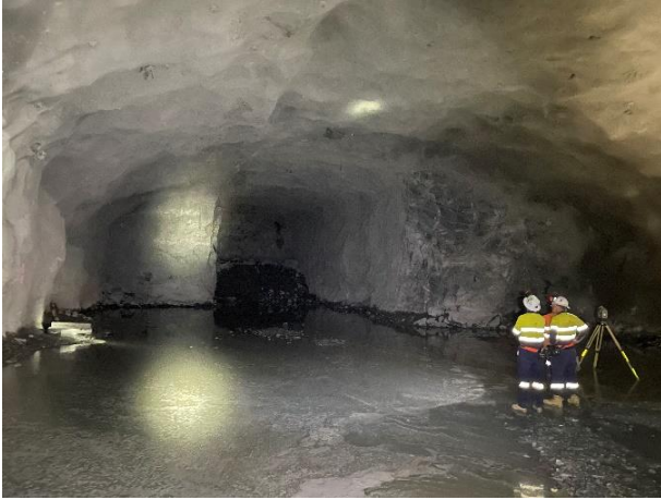
Figure 1: Power station cavern excavation
