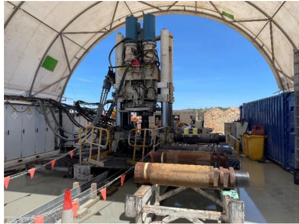
Figure 2: Raisebore Machine Excavating Ventilation Shaft
