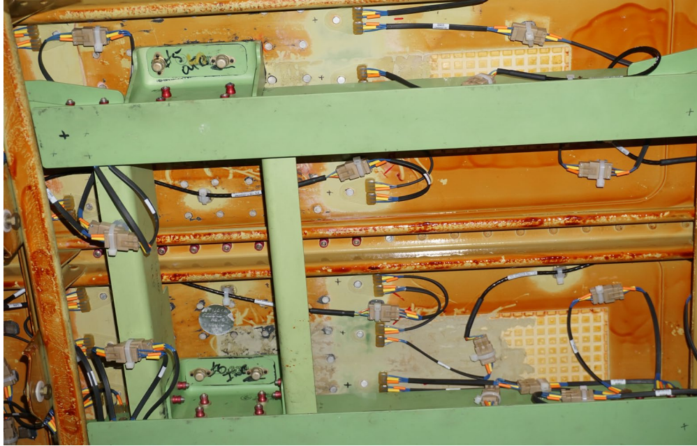
Figure 3. Looking u-Center of top crown of aircraft, sensors installed on critical fasteners
